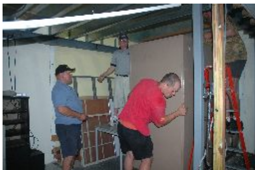
The improvements at the clubrooms are not happening by themselves. Here are the people making it happen.....
