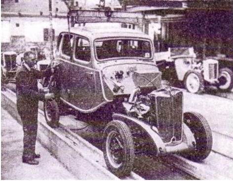
'Y' type saloons were assembled at Abingdon while 'TC' Midgets were still in production. However, most of the 'Y' chassis components later formed the basis of the 'TD' Midget.
